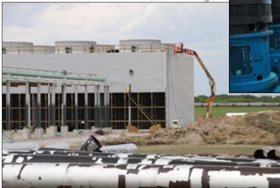
*Construction is nearing completion on the new cooling tower at Golden Grain Energy. Tying the tower into the rest of the plant will be the largest project undertaken during the annual shutdown June 20-24. The new tower will address quality and safety issues presented by steam with the previous cooling tower, in addition to meeting plant capacity.*
